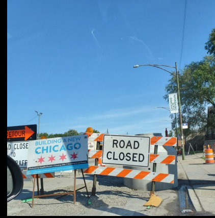
Construction on 87th Street
